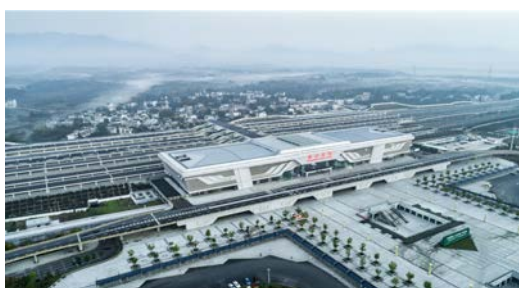
黄山高铁北站 Huangshan high-speed Railway North Station
